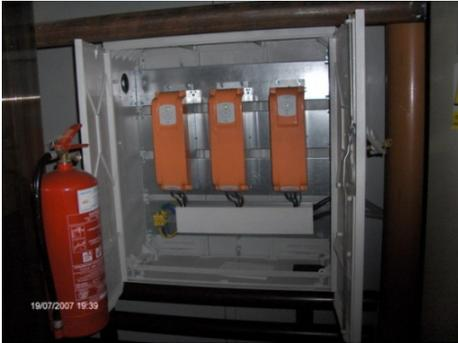
Lamps for external lighting. The LEC was effectively installed on both sets of lighting and saves approx. 21% of the utility bill for particular lighting circuits at this facility.
